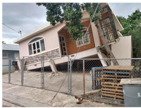
A house in southern Puerto Rico in the municipality of Guayama that was built upon stilts. The columns buckled during the shaking caused by the M 5.8 earthquake just offshore on January 6, 2020. This is a classic "soft first story" building. Photo credit: Fernando Martínez Torres.
