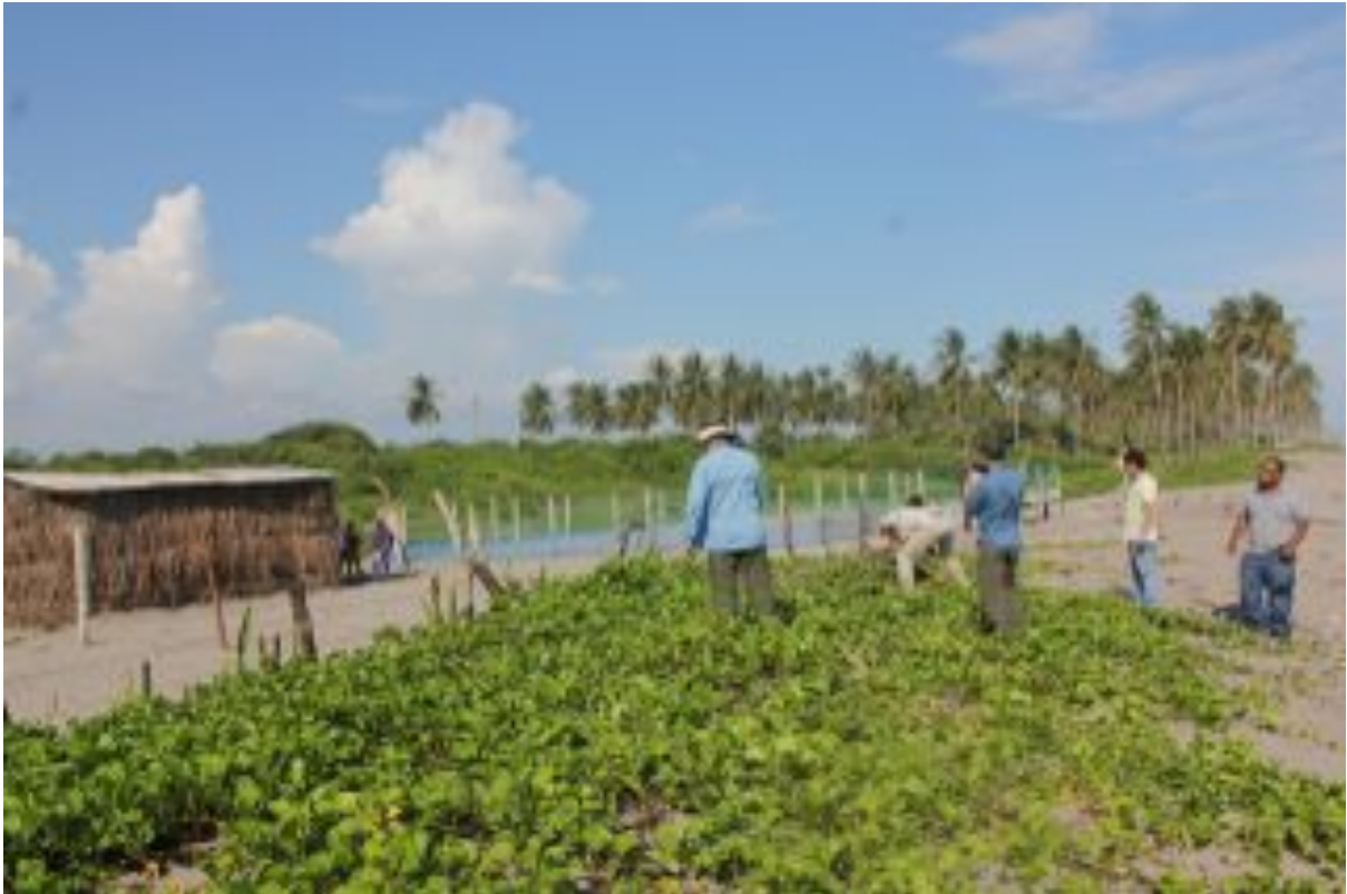
Figure 3.9 Corral de Mulas 2. The tsunami reportedly flowed over the beach dune but did not reach the hut in the back ground. No damage to the hut.
