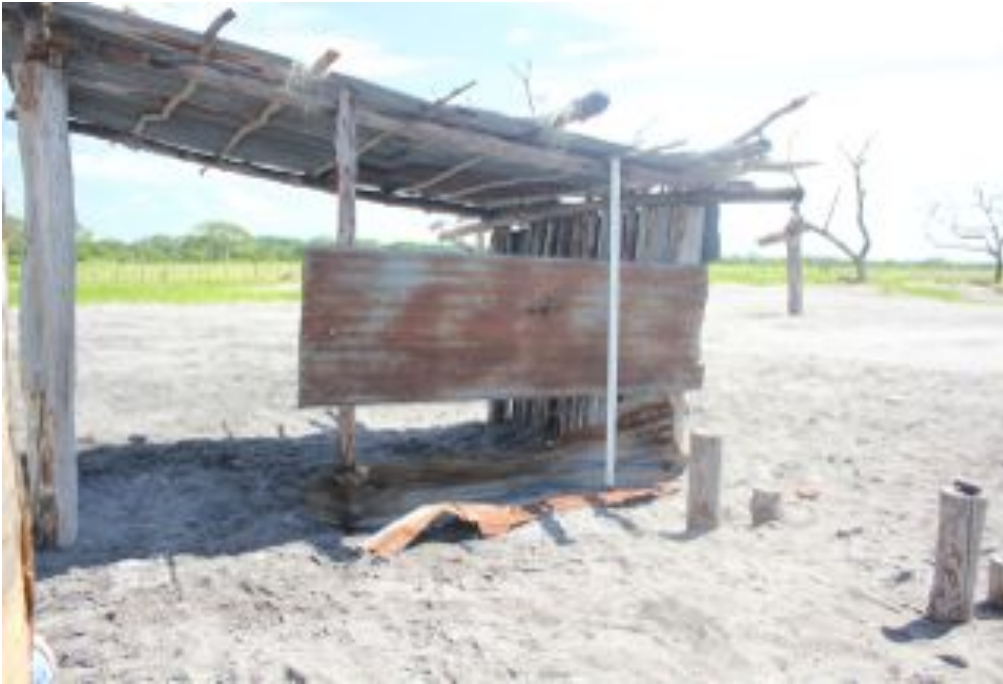
Figure 3.23 At the edge of the dead forest. Evidence of tsunami surge flowed under the intact piece of corrugated metal.
