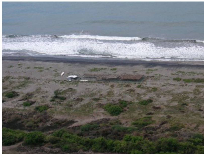
Figure 3.4. Aerial views of Isla de Mendez. The browning of the vegetation due to salt water penetration from the tsunami is evident. The structures had been rebuilt since the tsunami. The inundation extent is to the edge of the photo frame.
